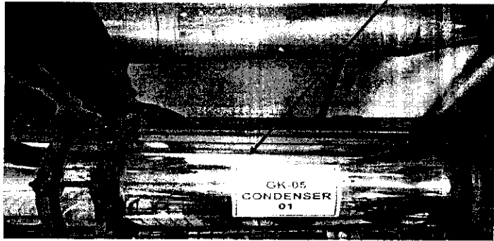
Horizontal primary condenser of GK-05
